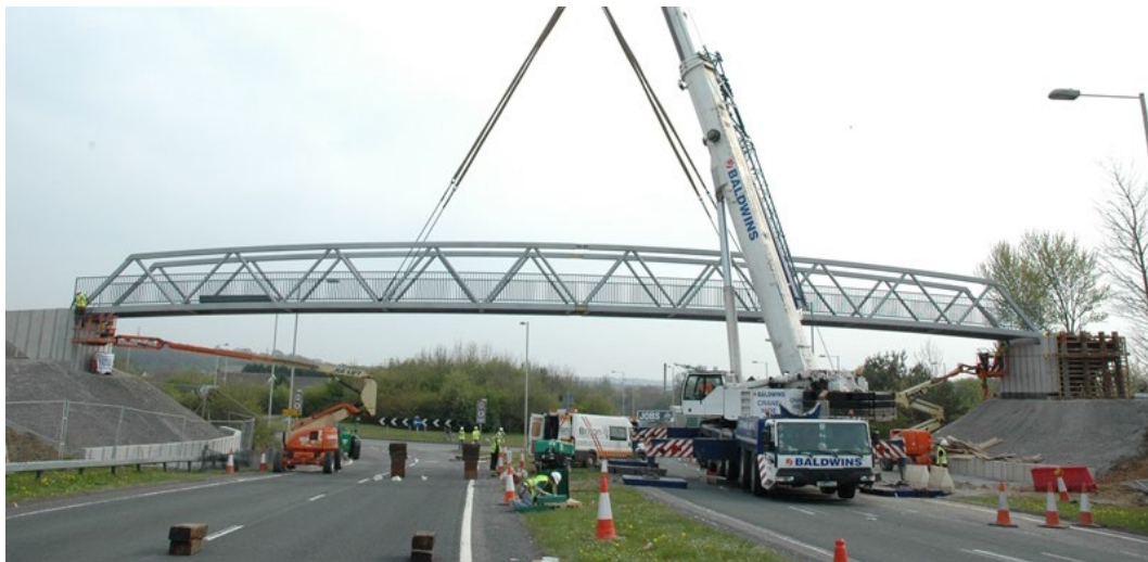
Figure 20: Bridge Erection during Road Closure
