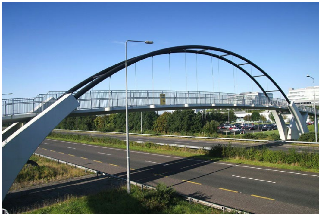
Figure 17: Shouldered Tied Arch Bridge Example – N19 Co. Clare
