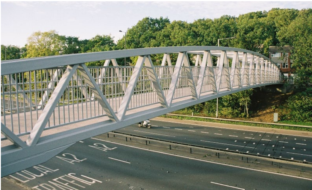
Figure 16: Single Span Through Girder – A2 Midhurst Warren Truss, UK
