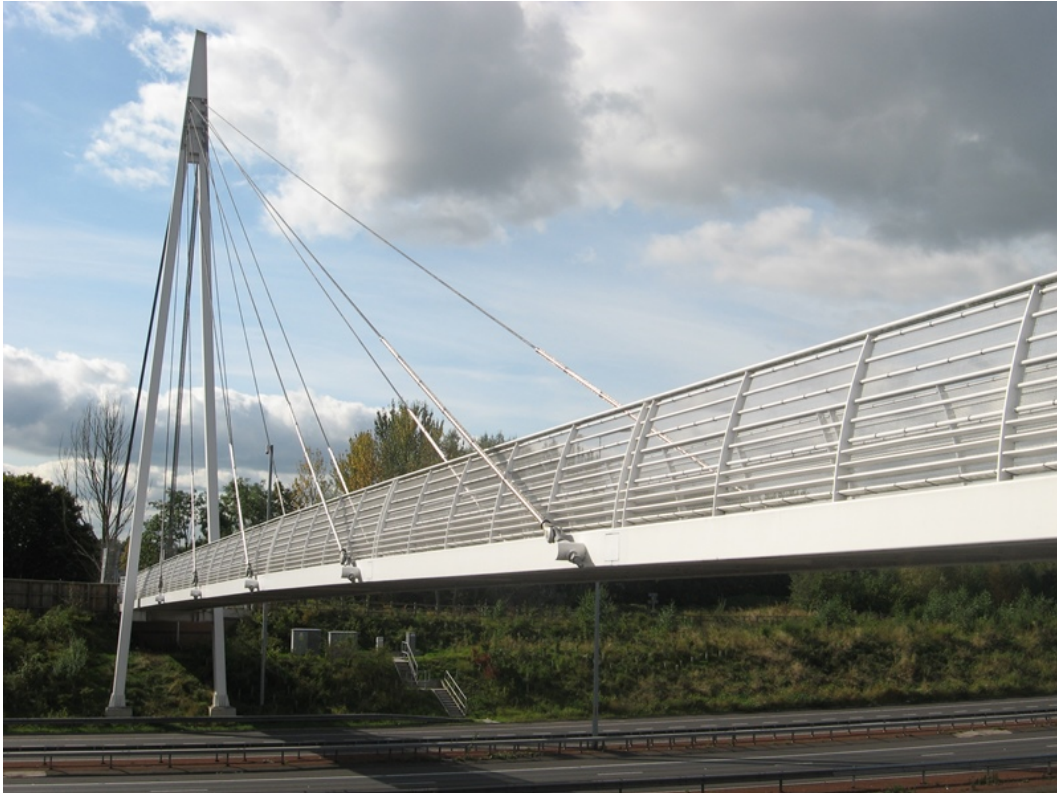
Figure 19 Cable Stayed Bridge Example
